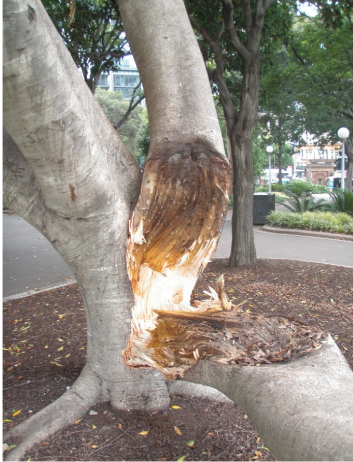
Image 4 – Hills Fig that had an included branch failure in Hyde Park South (adjacent to War Memorial).
